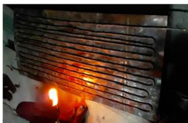
Fig. S8. Copper tube (3/8<sup>th</sup> inch diameter) being brazed on a 1.1 mm thick copper sheet of 1480 mm length × 660 mm width to prepare copper conduit attached to copper sheet.
