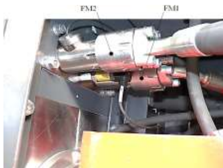
Figure 6: Flow meters FM1 and FM2 of the high-pressure lines of the test bench
