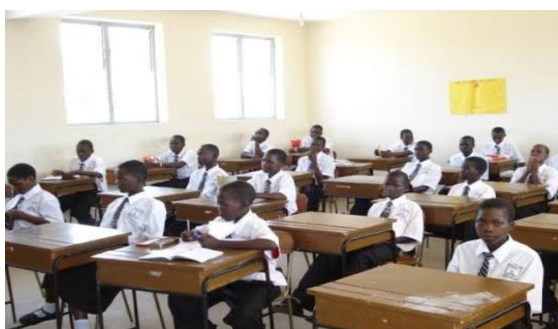
Plate 3: Condition of One of the Secondary Classrooms in Agege LGA.
